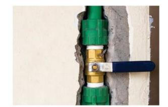
More over, PPR is characterized by its chemical resistance, high thermal resistance and good fatigue strength, PPR is of high molecular weight and is stabilized to high temperature, if corresponds to KTWrecommendation of the German Board of Health.
